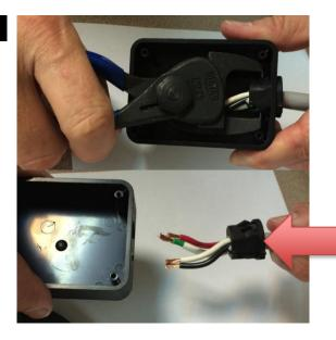
Remove the black strain relief with the enclosed strain relief pliers. Depress the tabs on the strain relief and remove the cable assembly from the plastic housing.
